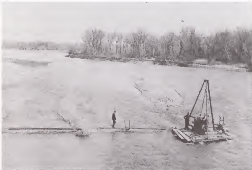
Core drilling rig for the Huntley Bridge on the Yellowstone River in 1944. (Photograph courtesy of Bob Robbins).
